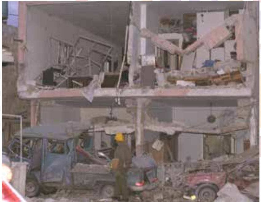
APARTMENT BUILDING DESTROYED BY A SCUD MISSILE.
