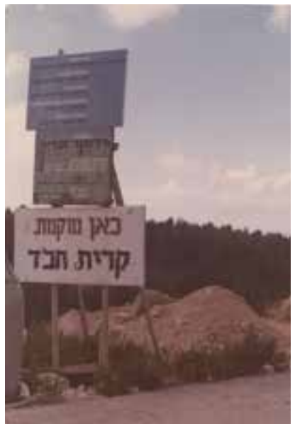
CONSTRUCTION OF THE KIRYA.
