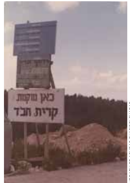
CONSTRUCTION OF THE KIRYA.
