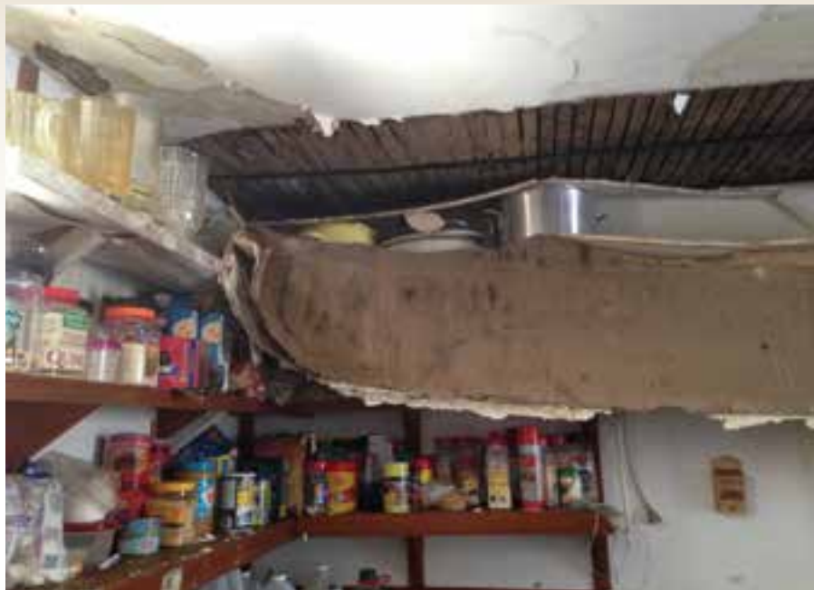
THE KITCHEN AFTER IT WAS FLOODED.
