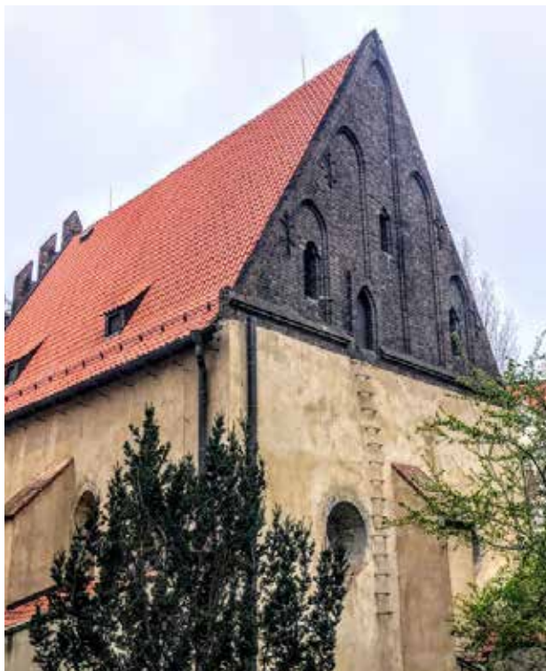
REAR OF THE THE ALTNEU SHUL, SHOWING RUNGS LEADING TO THE ATTIC WHERE THE REMAINS OF THE GOLEM ARE SAID TO HAVE BEEN STORED.
