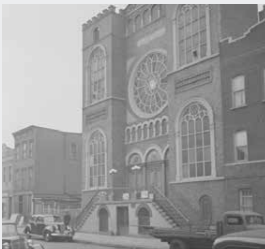
THE SHUL IN BROWNSVILLE WHERE THE FRIERDIKER REBBE DAVENED FOR THE YOMIM NORAIM, 5690.
