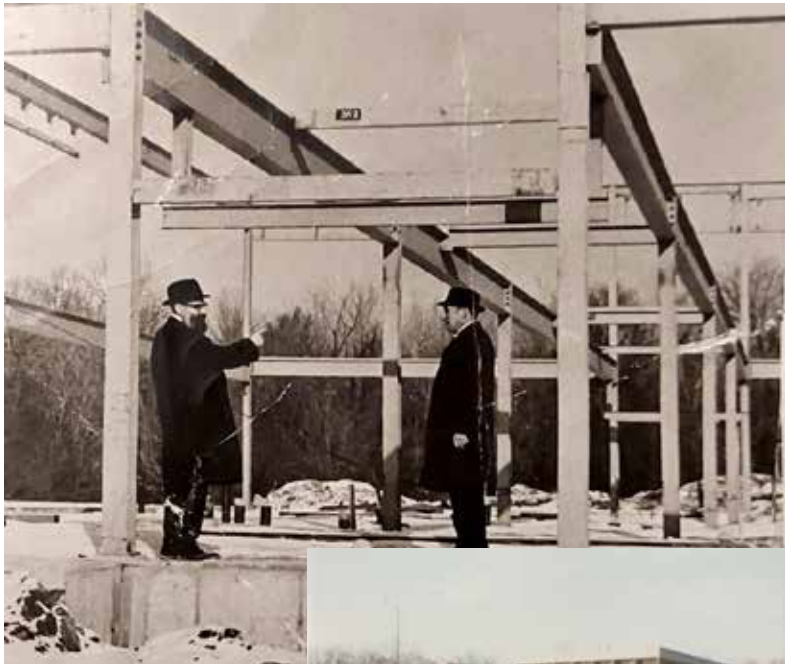
REB MOSHE YITZCHOK STANDS ON THE CONSTRUCTION SITE OF THE NEW BUILDING.
