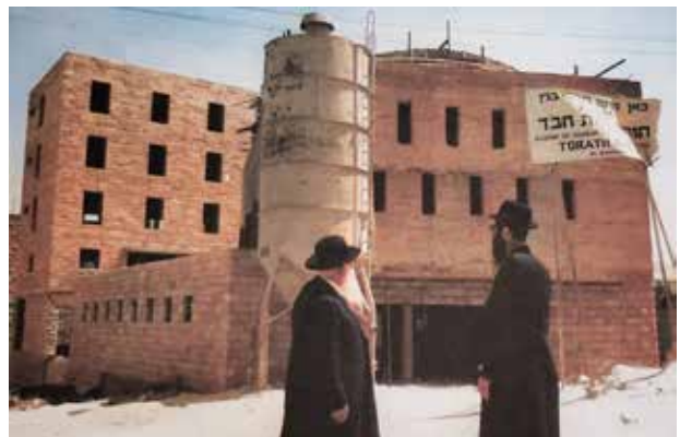
THE BUILDING DURING ITS CONSTRUCTION
