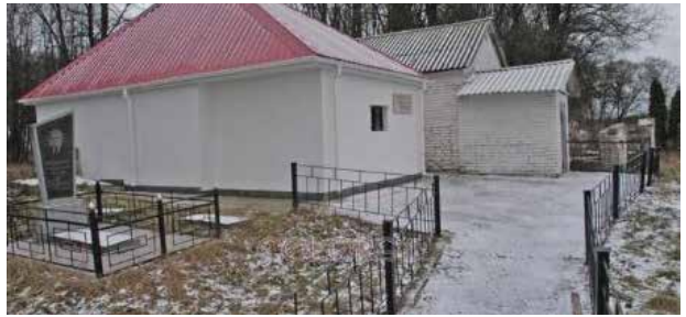
THE TZIYON AND SURROUNDING BUILDING TODAY, AFTER EXTENSIVE RENOVATIONS
