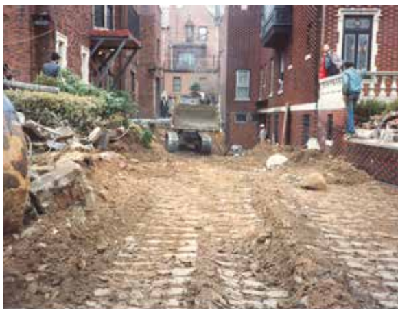
CONSTRUCTION TO EXPAND THE LIBRARY, 5750.
